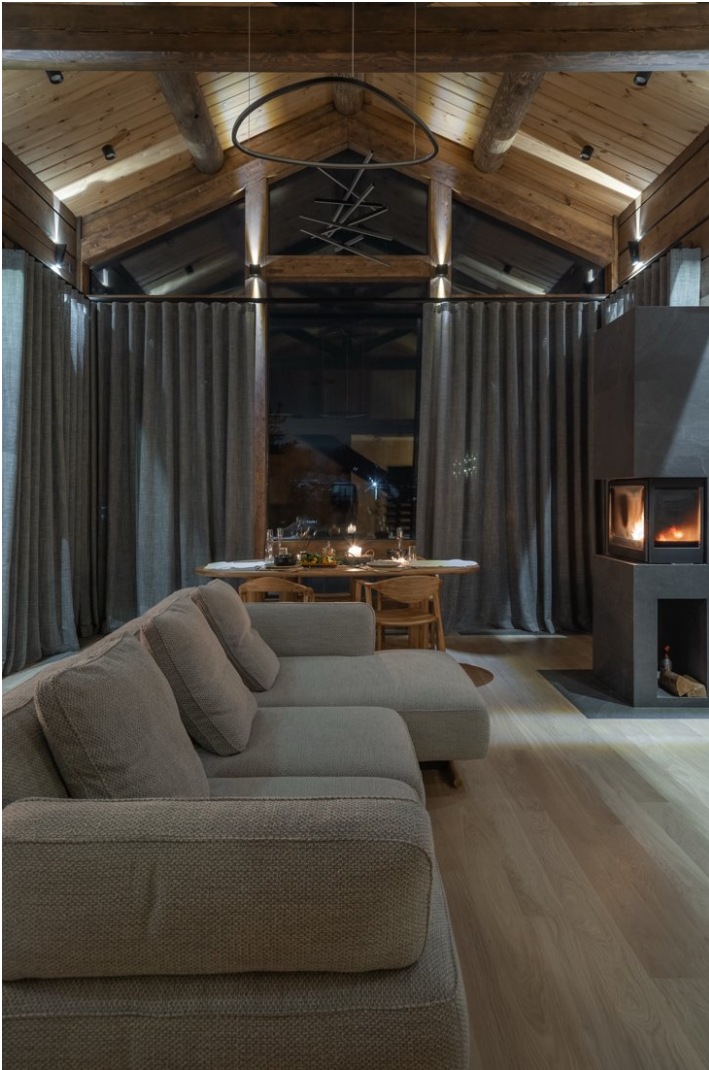
Timber roof structure with exposed purlins Exposed purlins, timber lining and integration of structure and space.
