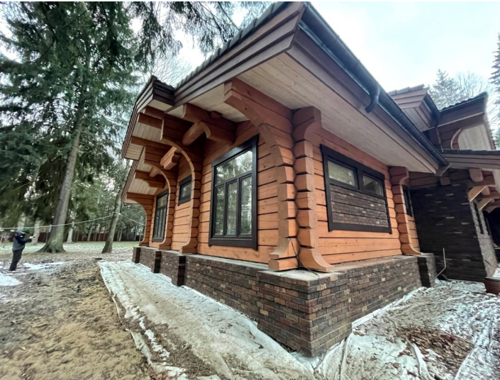
Assembled exterior corner of the log structure
