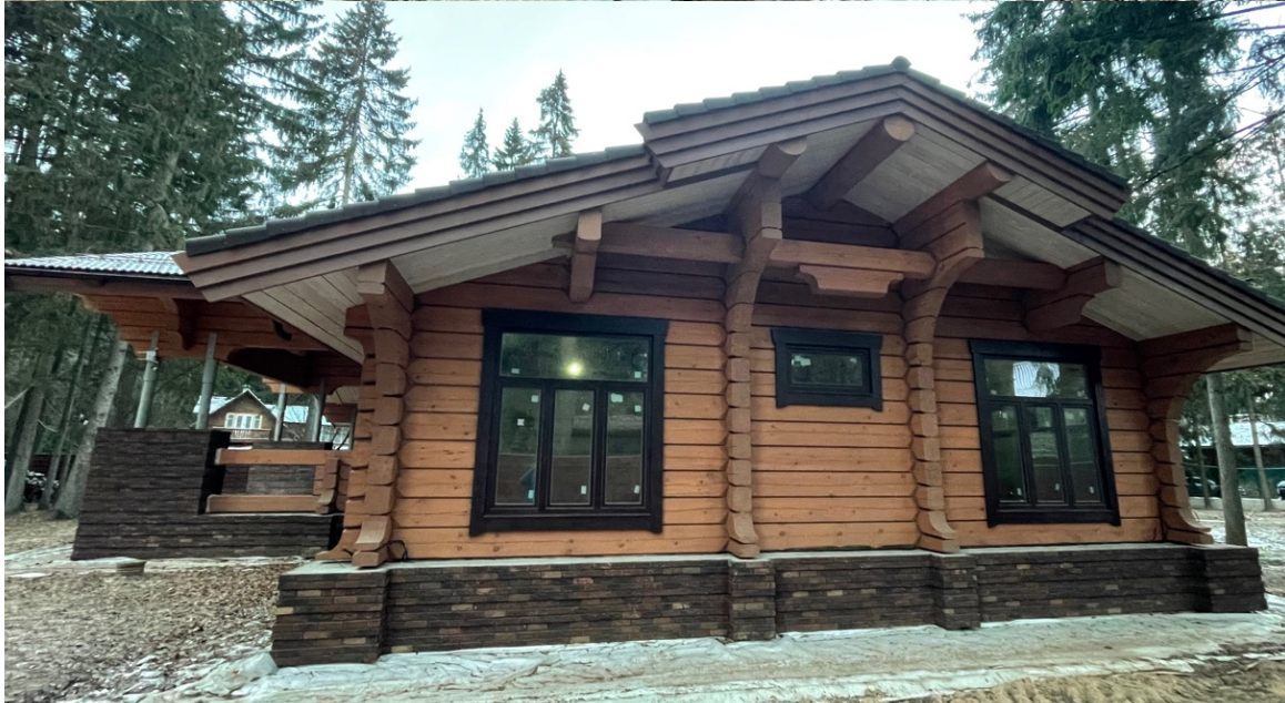
Flagship timber house, 700+ m 2 Large-scale bespoke timber house constructed from kiln-dried timber beams measuring 250 × 350 mm.
