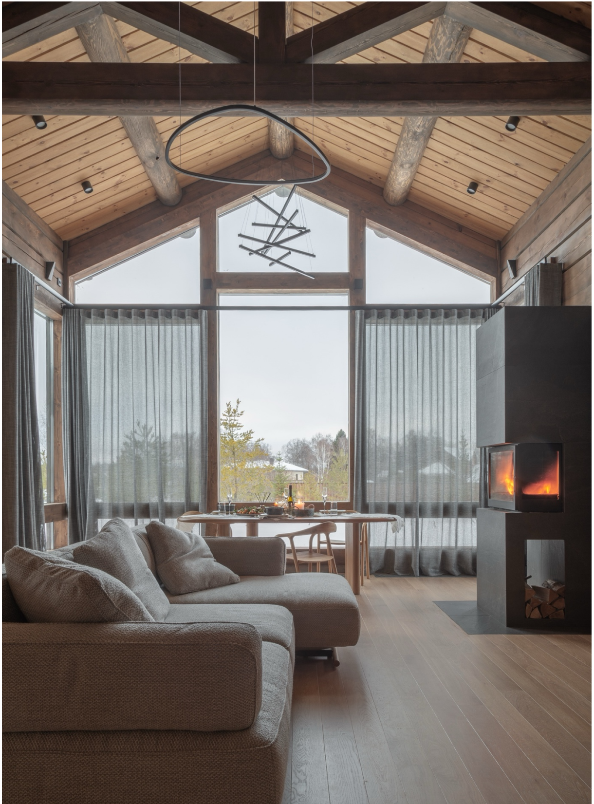
Timber roof structure with exposed purlins Interior roof structure showing exposed purlins, timber lining, and the integration of structural and spatial expression.
