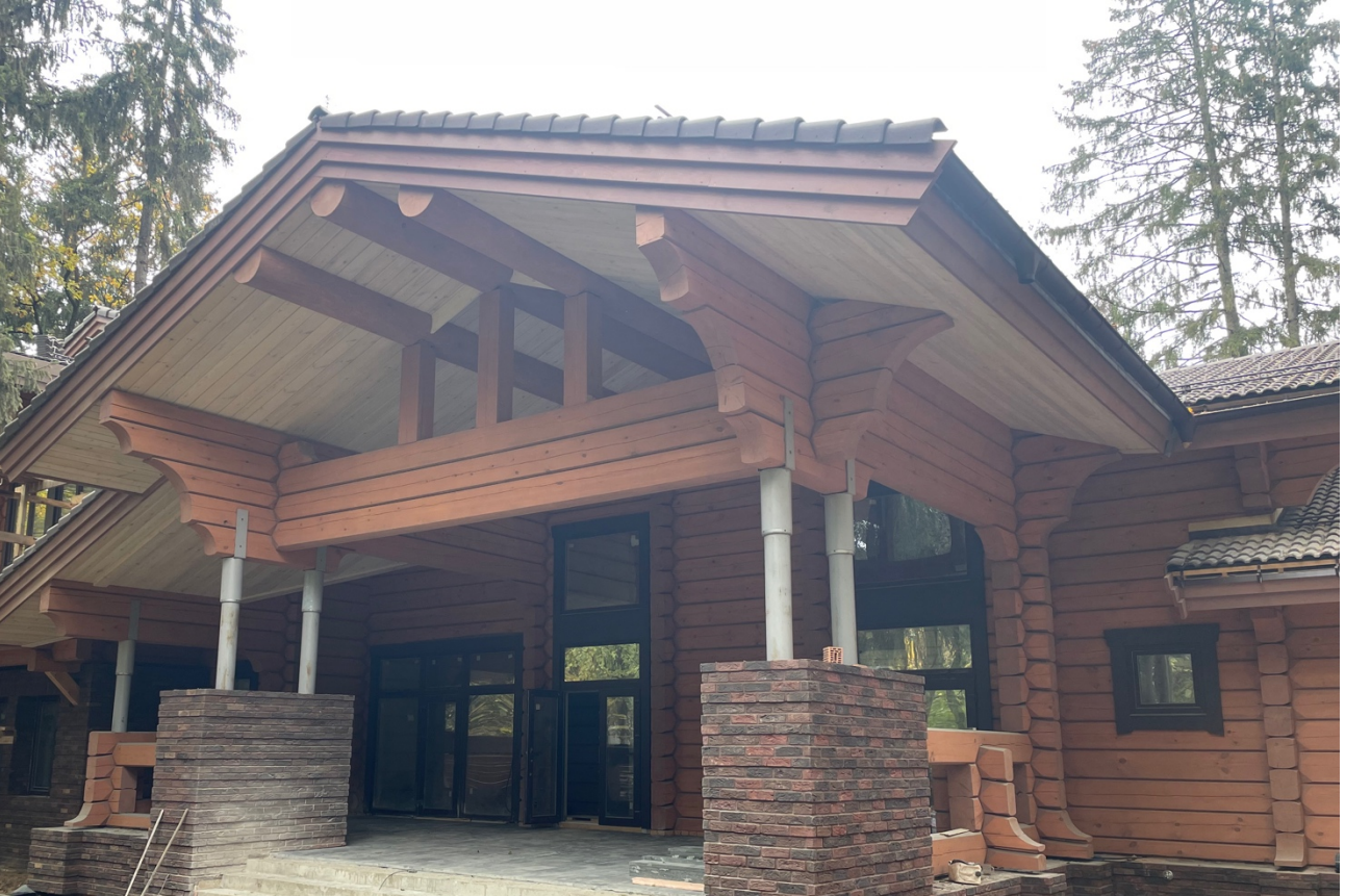
Roof ridge exceeding 9 metres Large timber roof structure with a ridge height exceeding 9 metres.
